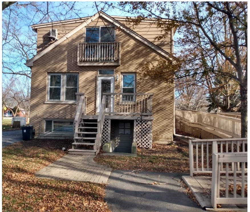
Right Image: Rear/west structure elevation.
